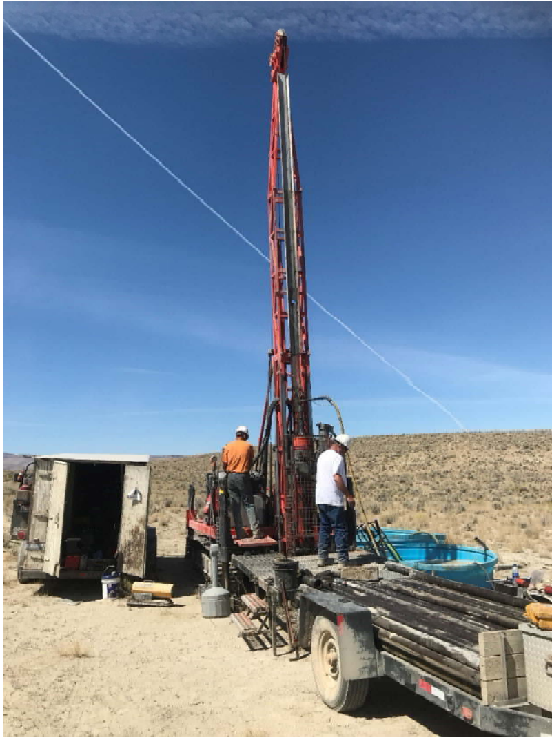
Figure 3 – Core drilling at McDermitt
